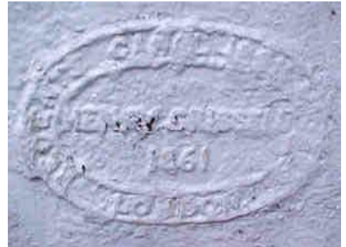
A maker's plate 1861 - Henry Grissell, Regents Canal Ironworks London OS ref: TL 271 035
